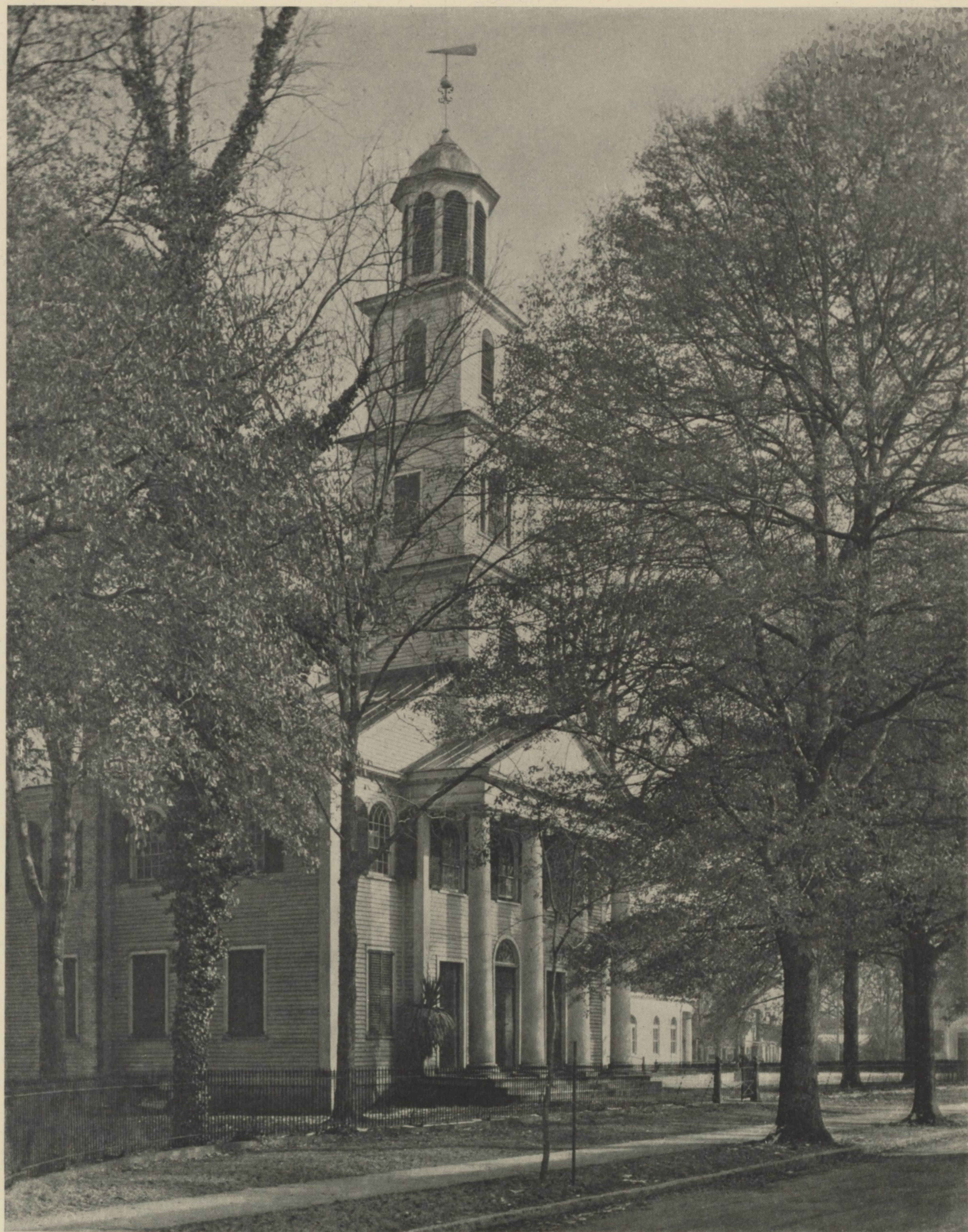
THE PRESBYTERIAN CHURCH, NEW BERN, NORTH CAROLINA
