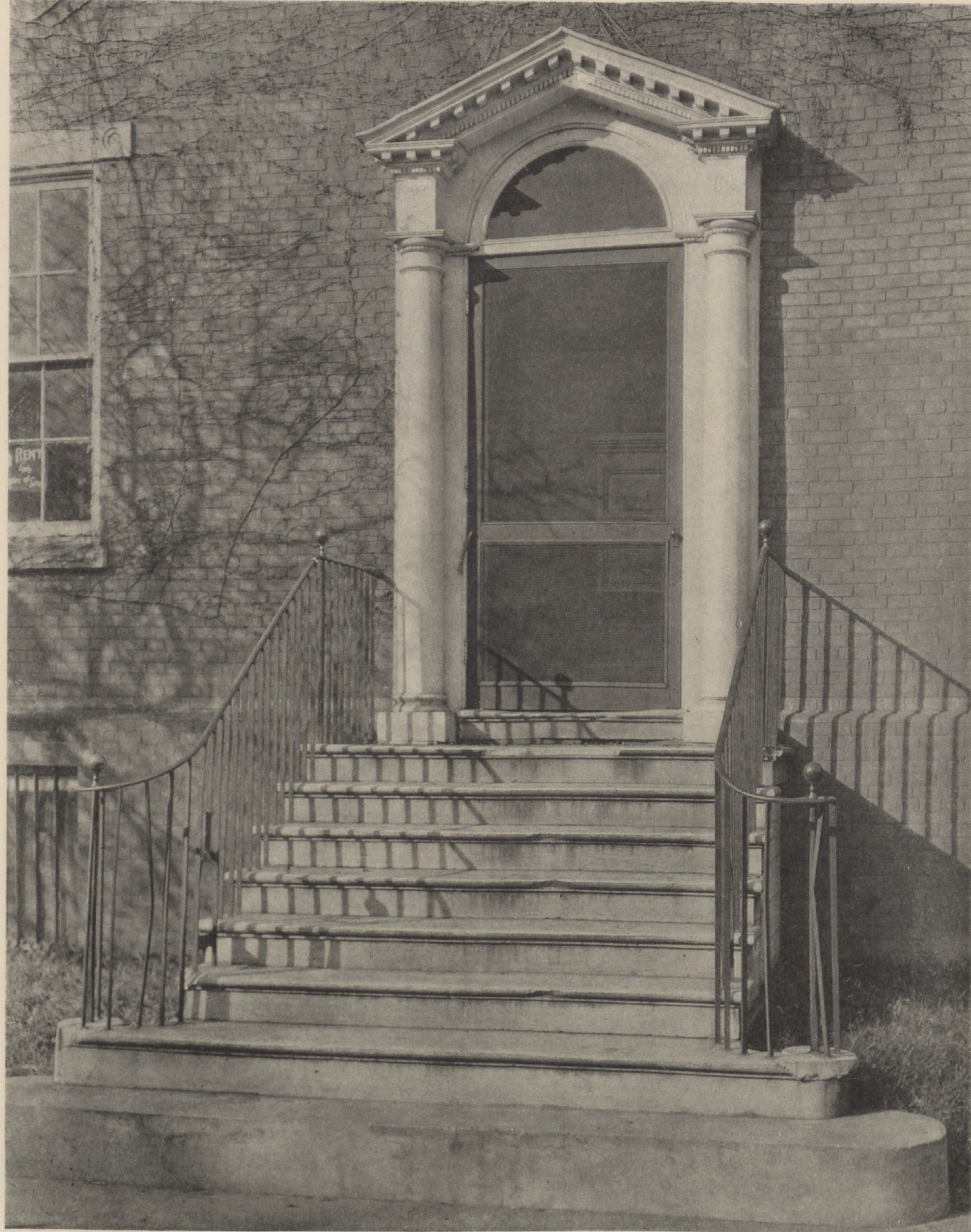
THE HUGHES HOUSE, CRAVEN STREET, NEW BERN, NORTH CAROLINA Torn down in 1925 and replaced by a garage!
