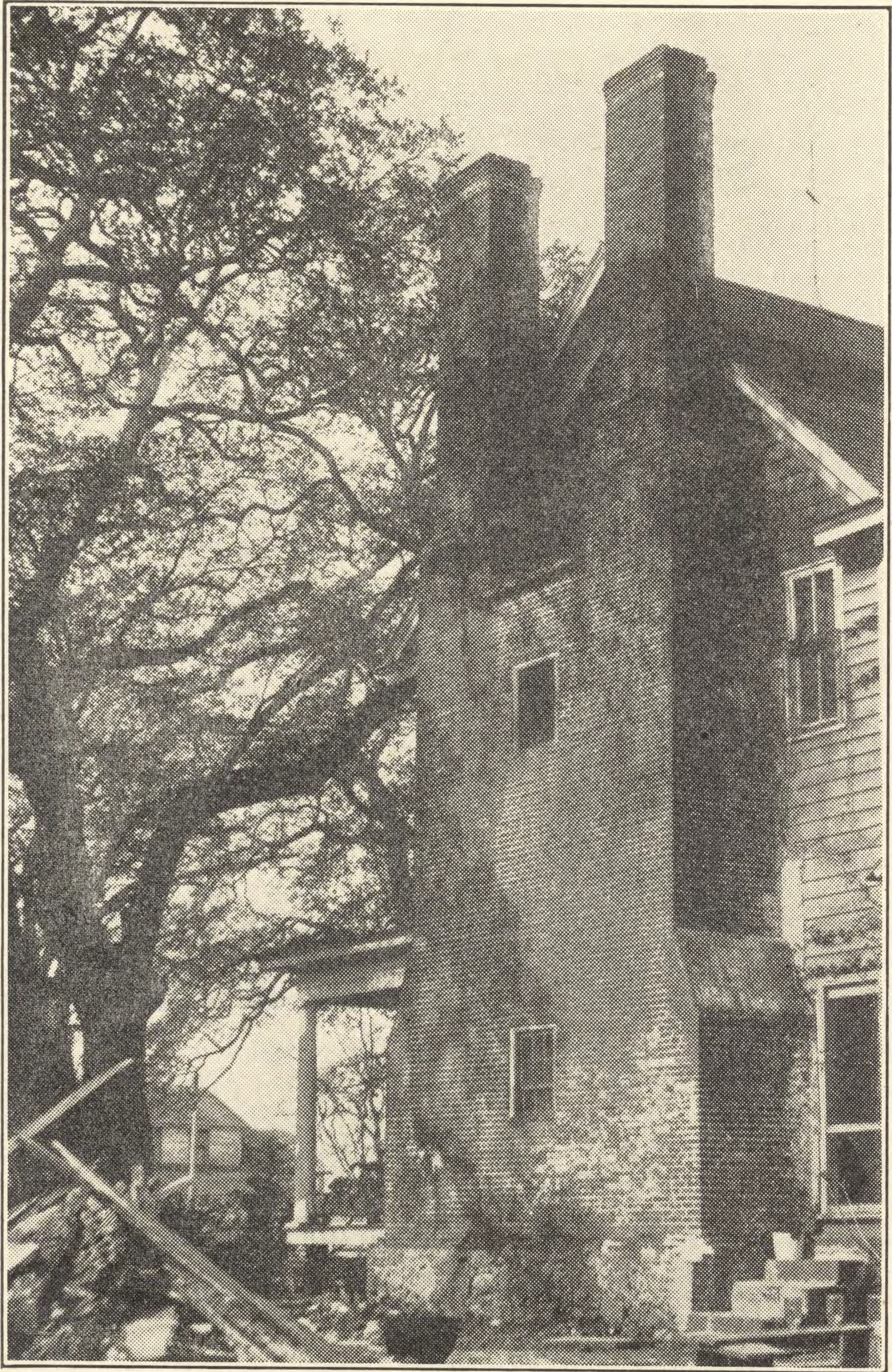
THE CHIMNEYS OF THE OLD MARSH HOUSE IN BATH BUILT 1744
