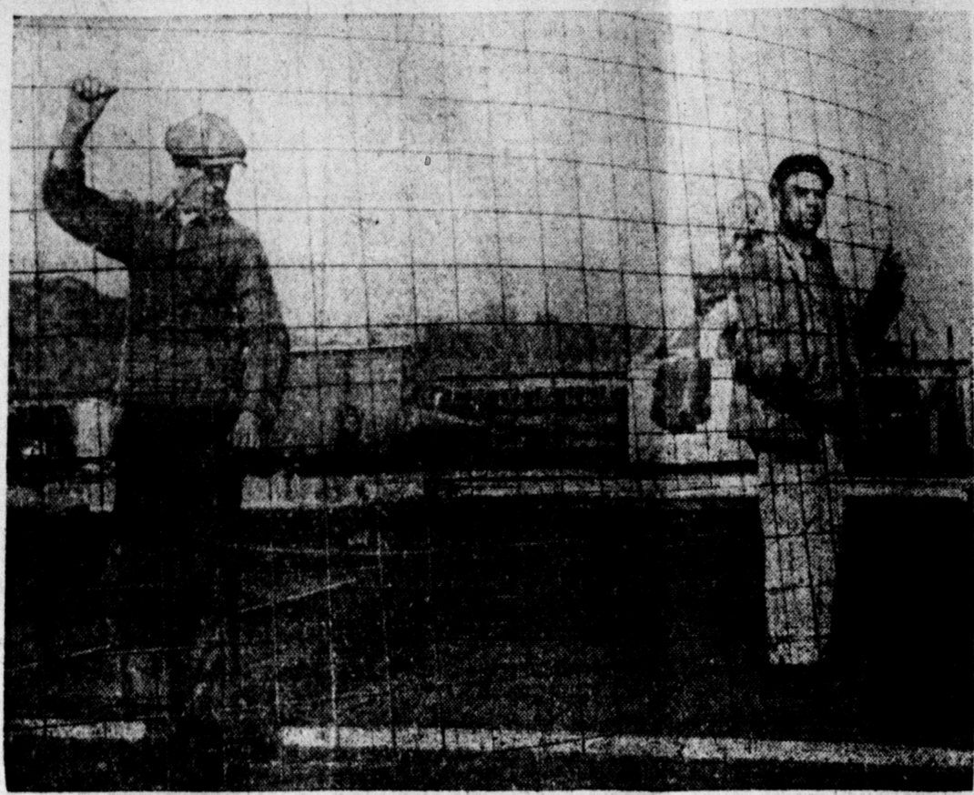
Strength For Heavy Load—Workmen Imbed Steel Mesh In New German 'Autobahn'
