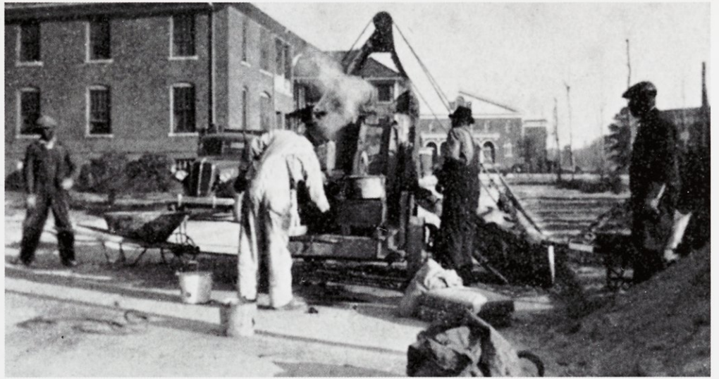
ABOVE: The campus revived in the decade with a well-plotted, curbed set of hardtop roadways. This crew is laying concrete behind Austin and neighboring residence halls. Works Progress Administration funds from the New Deal made the improvement possible.
