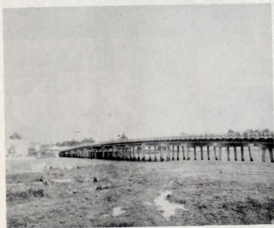
The New Scuppernong Bridge
