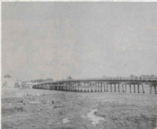
The New Scuppernon Bridge
