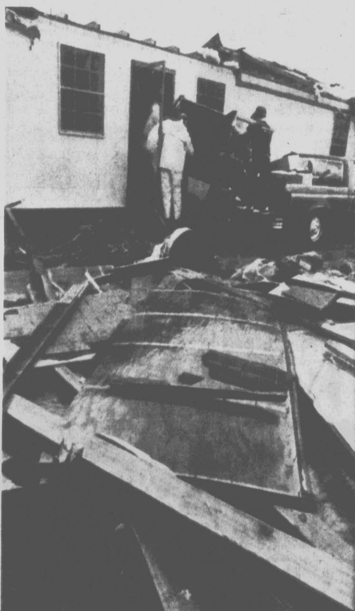
STORM DAMAGE — Neighbors help Carl East of LaBelle, Texas, remove belongings from his home Thursday after the roof was ripped off by Hurricane Bonnie. Gulf Coast residents are returning to their homes after the storm moved inland, leaving two people dead. (AP Laserphoto)
