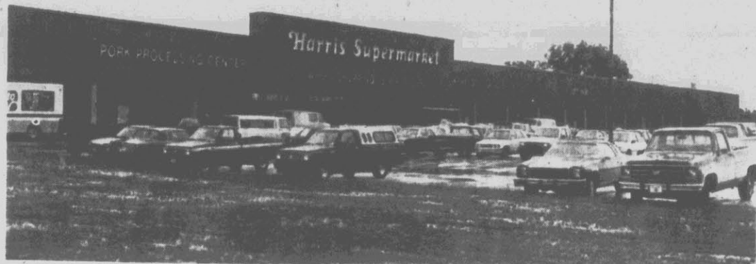
OPENING WEDNESDAY — This new Harris Supermarket, the anchor for the Bells Fork Square shopping center on N.C. 43 south, will open Wednesday. Ribbon-cutting ceremonies are scheduled for 11 a.m. The 40,000
