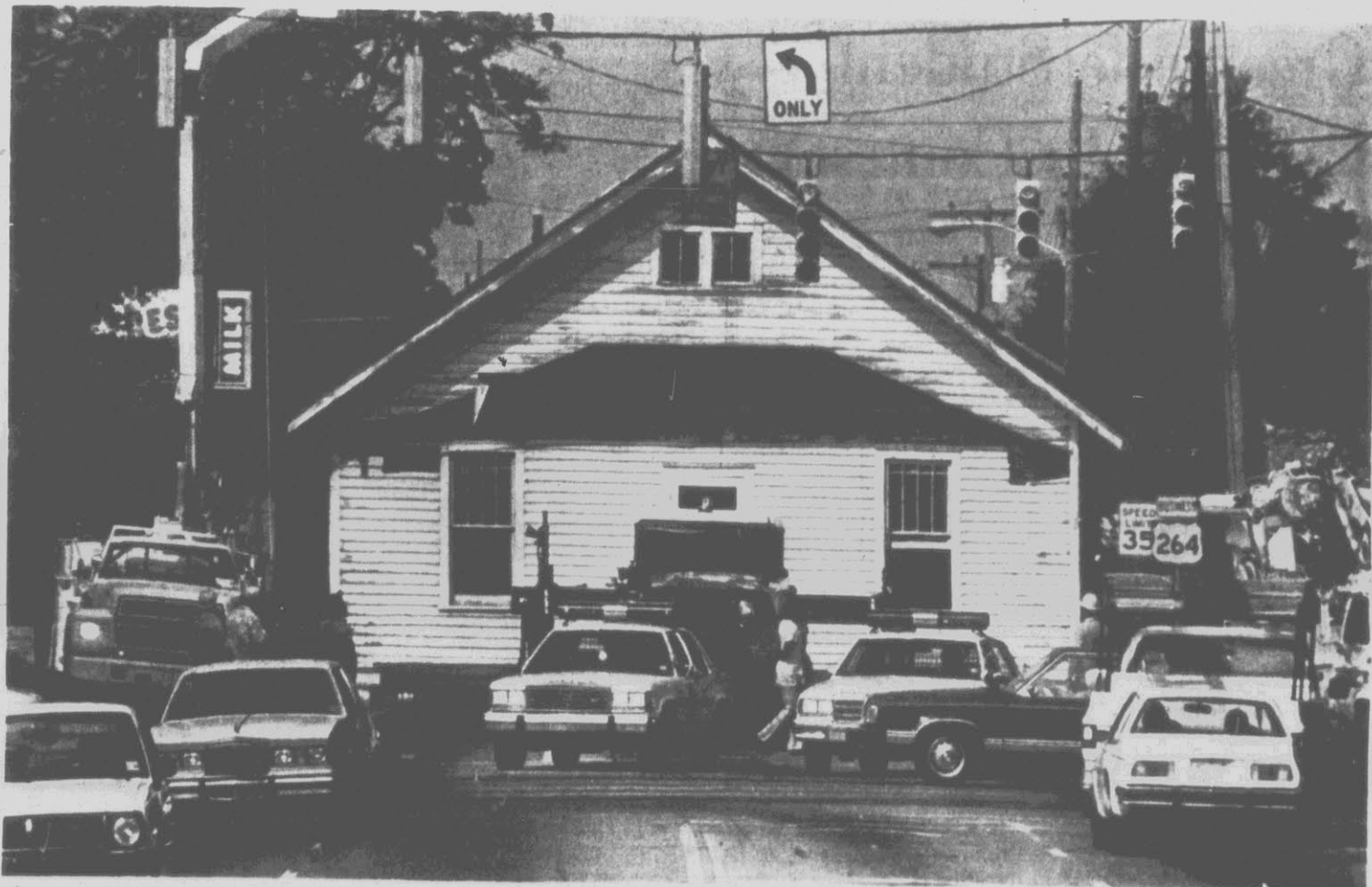
CAUGHT IN TRAFFIC — Employees of Barfield House Movers of Farmville slip a large house through traffic at 14th Street and Dickinson Avenue Monday morning. Most motorists made the proper detours, but there were times when the house seemed to move with traffic, stopping for traffic lights
