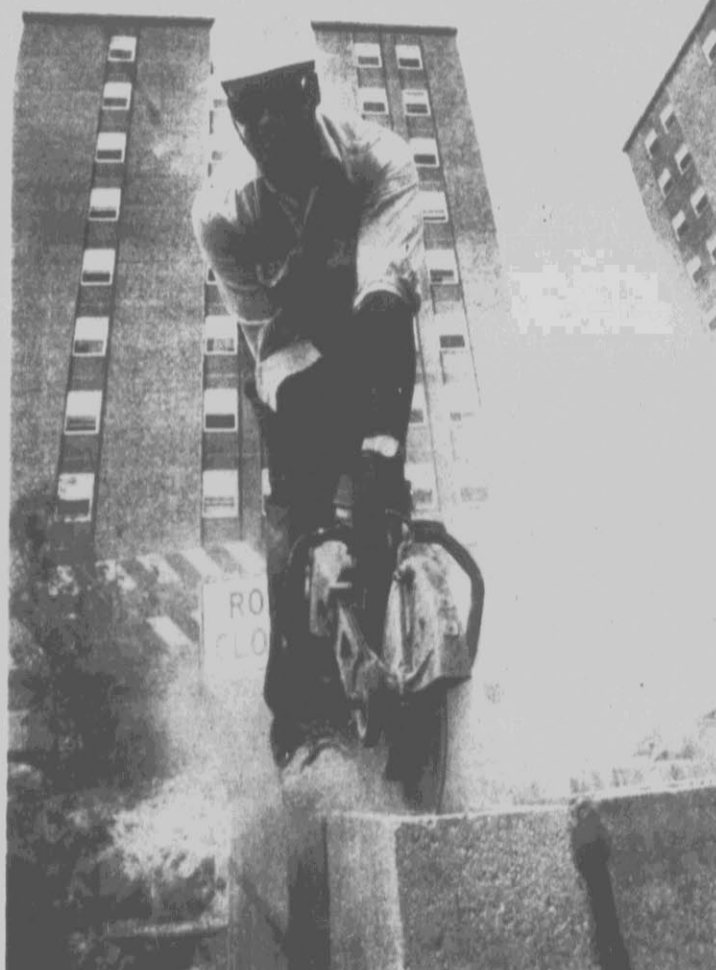
A HOT JOB — Lee Johnson, a Greenville Utilities Commission employee, saws grooves into concrete blocks for bracing. Johnson was with a crew of GUC workers putting in a new concrete vault for water valves at the corner of Reade and Charles streets. The crew worked through the summery temperatures Thursday afternoon. (Reflector Photo by Cliff Hollis)
