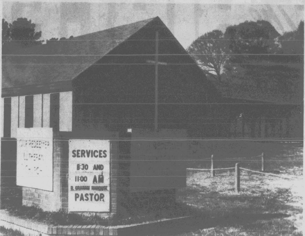
DEDICATION — A 3,200-square-foot sanctuary at Our Redeemer Lutheran Church will be dedicated at 4 p.m. Sunday. The facility will also house administrative offices. A Japanese style prayer garden is located behind
