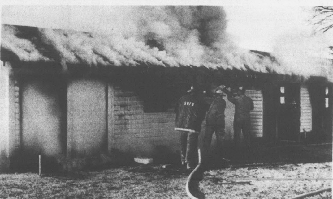
SHOP BURNS ... in a mid-afternoon fire yesterday at the Department of Corrections, Division of Prisons on the Belvoir highway. Above firemen try to gain entrance into the building. (Reflector Photo by Tommy Forrest)
