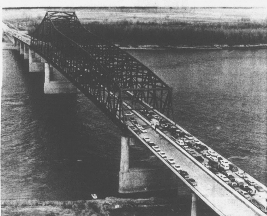
A DREAM OF 30 YEARS — Cars lined up Wednesday to be among the first to cross the new $77 million bridge linking Tennessee with the Missouri bootheel. The new bridge, sought by Missouri and
