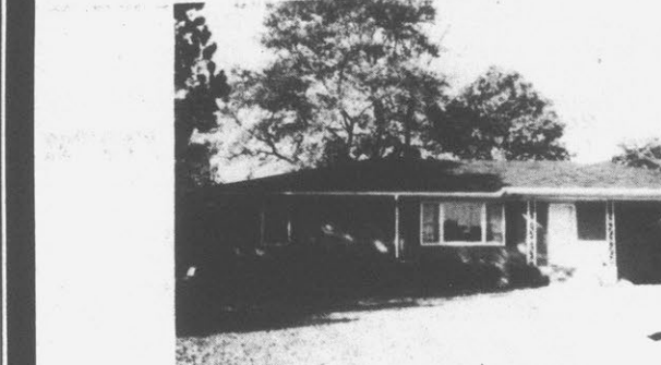
This brick home is convenient to school and shopping. It has 3 bedrooms, 1 1/2 baths, living room, new roof, new furnace, new central air, all at a price you can afford. Most important feature is the one full year home warranty offered only through ERA (Electronic Realty Associates) $33,500
