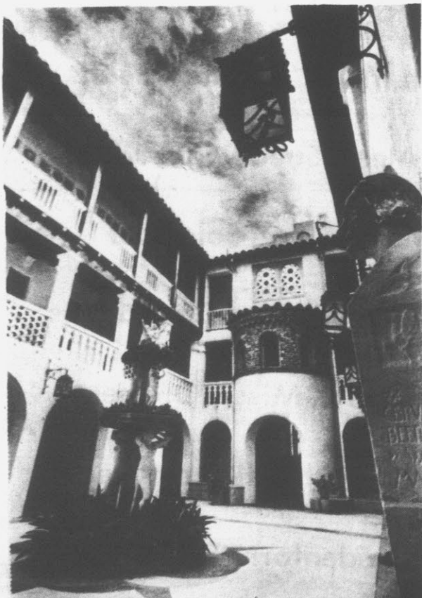
PRESERVING ART DECO — Designers and laymen are getting together to preserve the Art Deco and Mediterranean style hotels from the city of Miami's early days. The Amsterdam Palace, which was built in 1930 under the name of Casa Casuarina, is one being fixed up; hoping to bring back some of the excitement of the old days which many tourists on the beach remember well. (AP Wirephoto)
