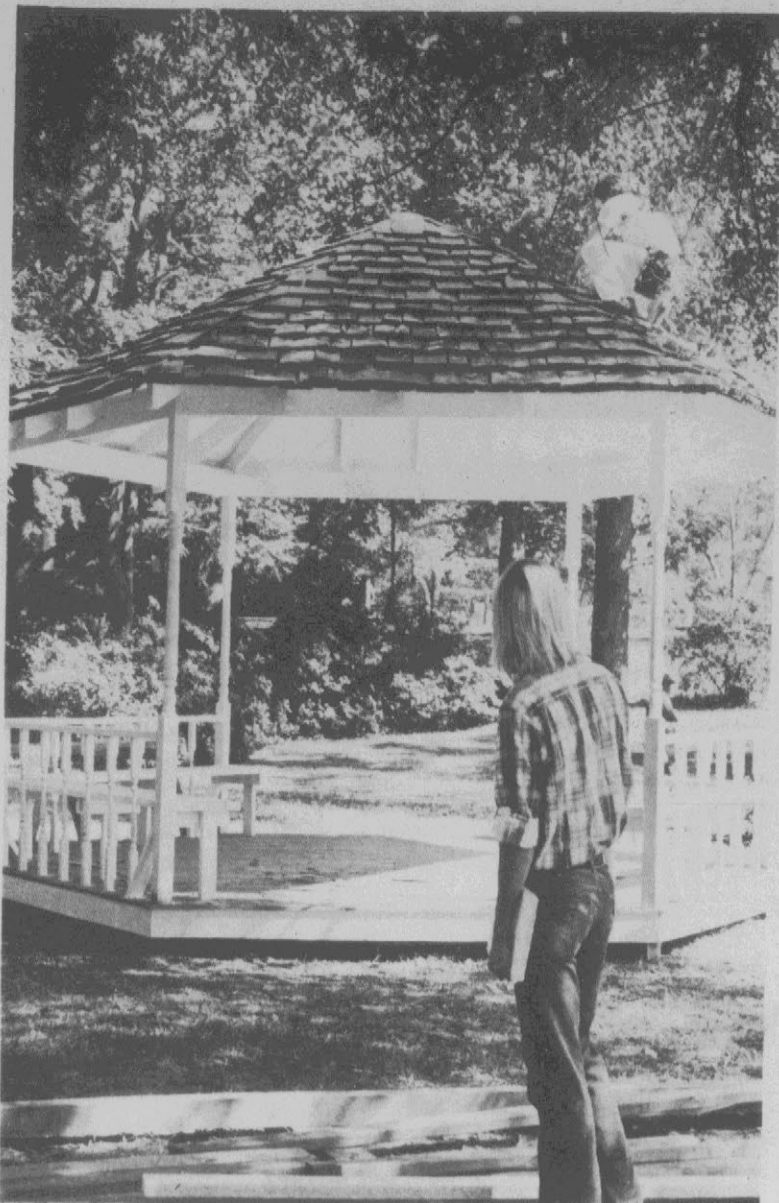
GAZEBO—An East Carolina University student pauses to look as Bill Dill, an ECU graduate from New Bern, clambers atop the gazebo he has designed and built in a special beauty spot on campus. The structure, gift of the Class of '74, will be finished as soon as Dill adds a few more shingles and last minute touches. (ECU News Bureau Photo by Marianne Baines.)
