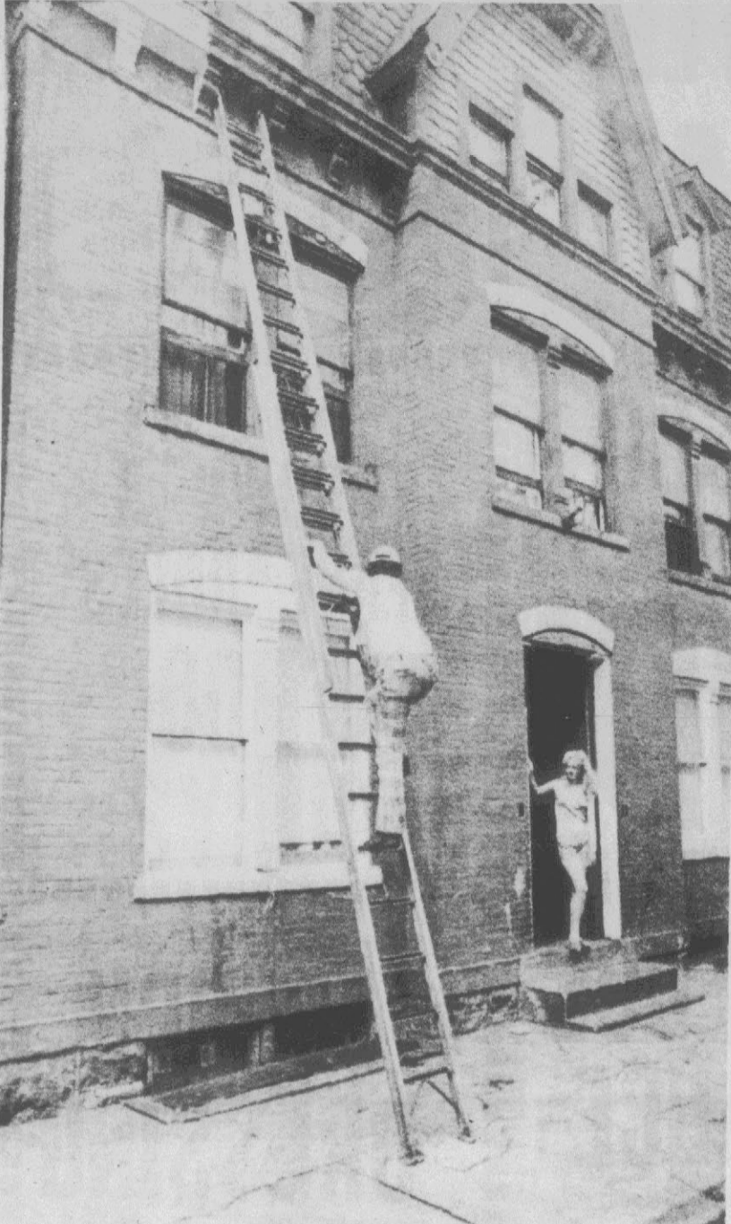
URBAN DECAY almost robbed Pittsburgh of one of its most fashionable and historic neighborhoods. Here a worker climbs ladder to do restoration job on upper floors of a building. (UPI Photo)
