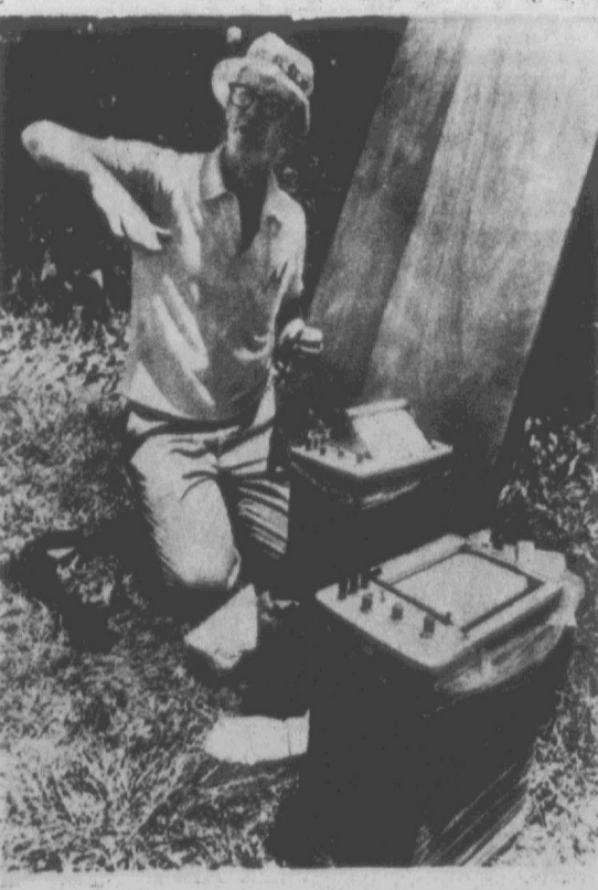
HOW IT WORKS —Scientist Francis G. West of the University of California's Los Alamos, N.M. laboratory, explains how a tiltmeter works, prior to installing the devices on the slopes of Guadeloupe's La Soufriere volcano. The instruments record any unusual ground changes which could help predict an eruption. (AP Wirephoto)
