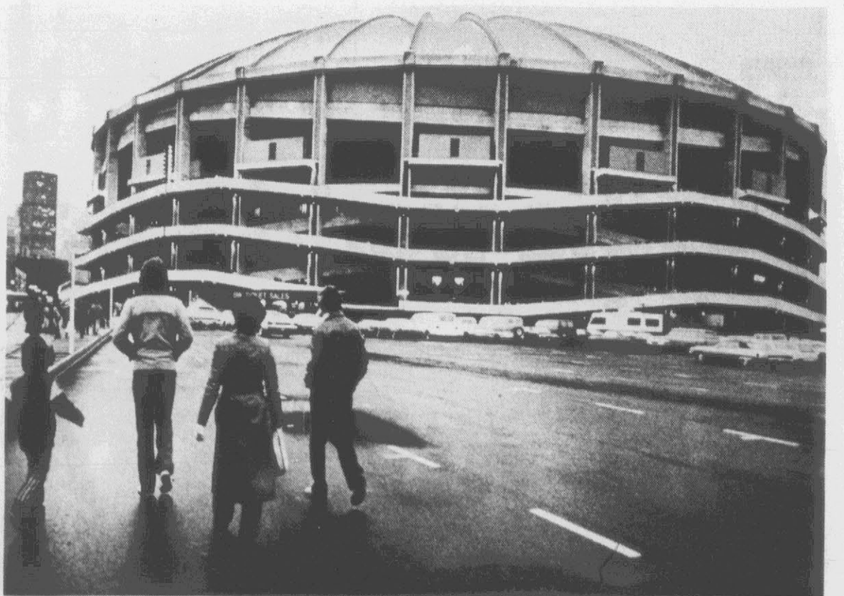
Now in business: King County Domed Stadium, new object of civic pride for Seattle.
