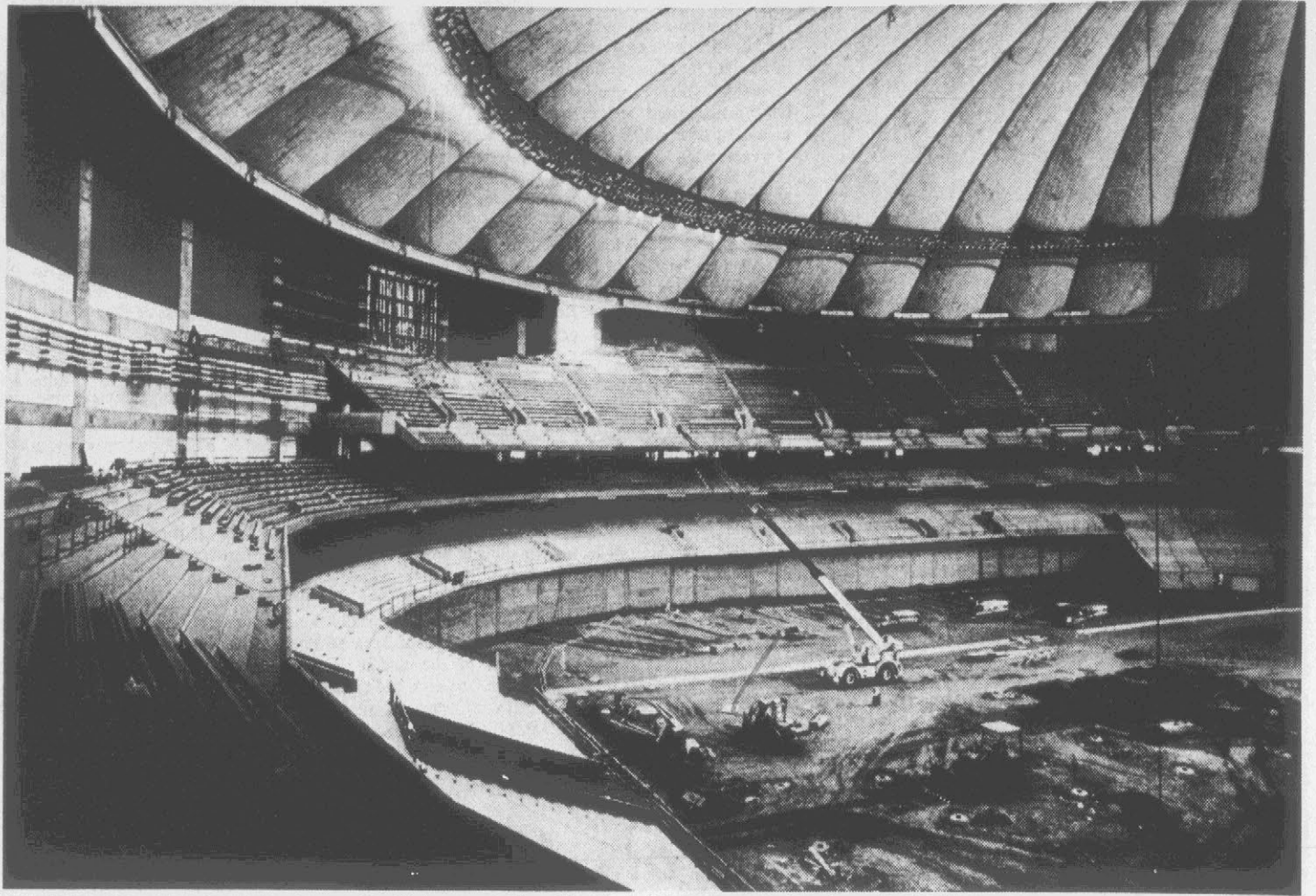
Seattle's new stadium dwarfs building crews and equipment.
