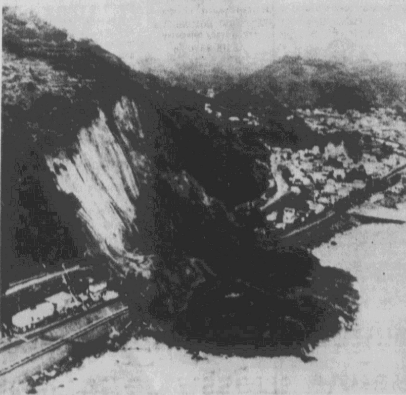
LANDSLIDE — A side of a hill in Shimoda, Japan, covers railway tracks and houses after a landslide took place in the town, south of Tokyo, Sunday. Nine people were reported killed and about 30 homes destroyed. (AP Wirephoto)
