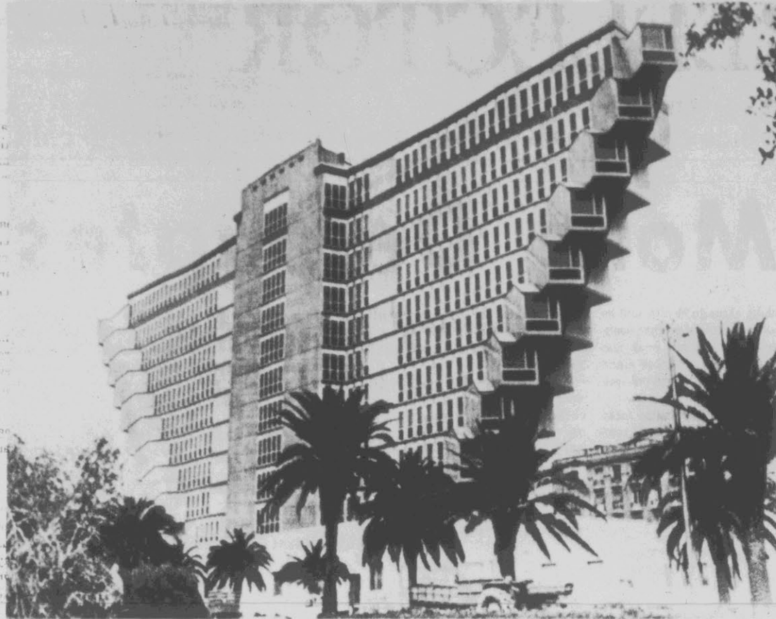
THE MODERN LOOK — The Hotel du Lac, in the heart of Tunis, Tunisia, displays a somewhat unorthodox architectural design. The upside-down look features rooms hanging at the end of each wing of the structure.
