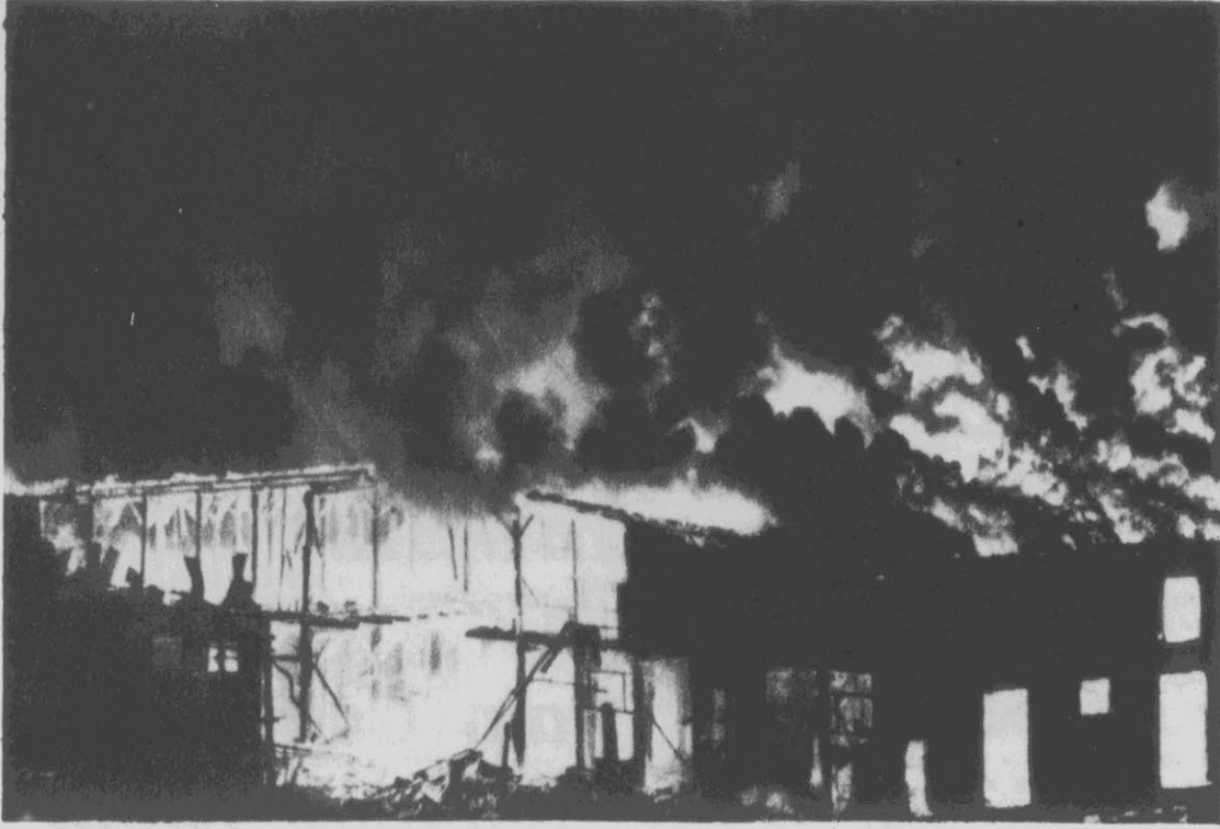
FIRE ON THE WATERFRONT —Flames and massive columns of smoke range through a gutted Conrall pier on the Hudson River late Thursday night as the fire broke out in an area full of abandoned wooden shacks and piers in Weehawken, N. J. The flames lit up the New Jersey waterfront and the west side of New York City across the river. (AP Wirephoto)
