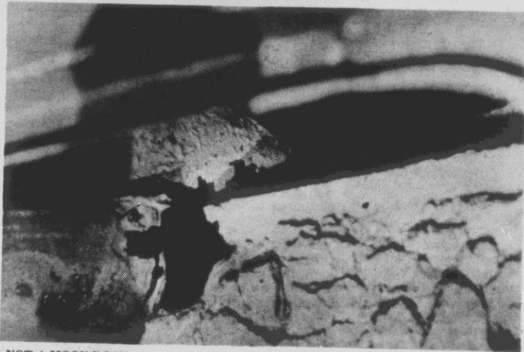
NOT A MOON ROCK sample but a close-up of body damage on a car. According to the Windsor, Ontario, Police, damage such as this rates high among the safety defects they have discovered in safety checks. Such damage is dangerous because the protective shell the car builds around passengers is hampered in case of accidents.
