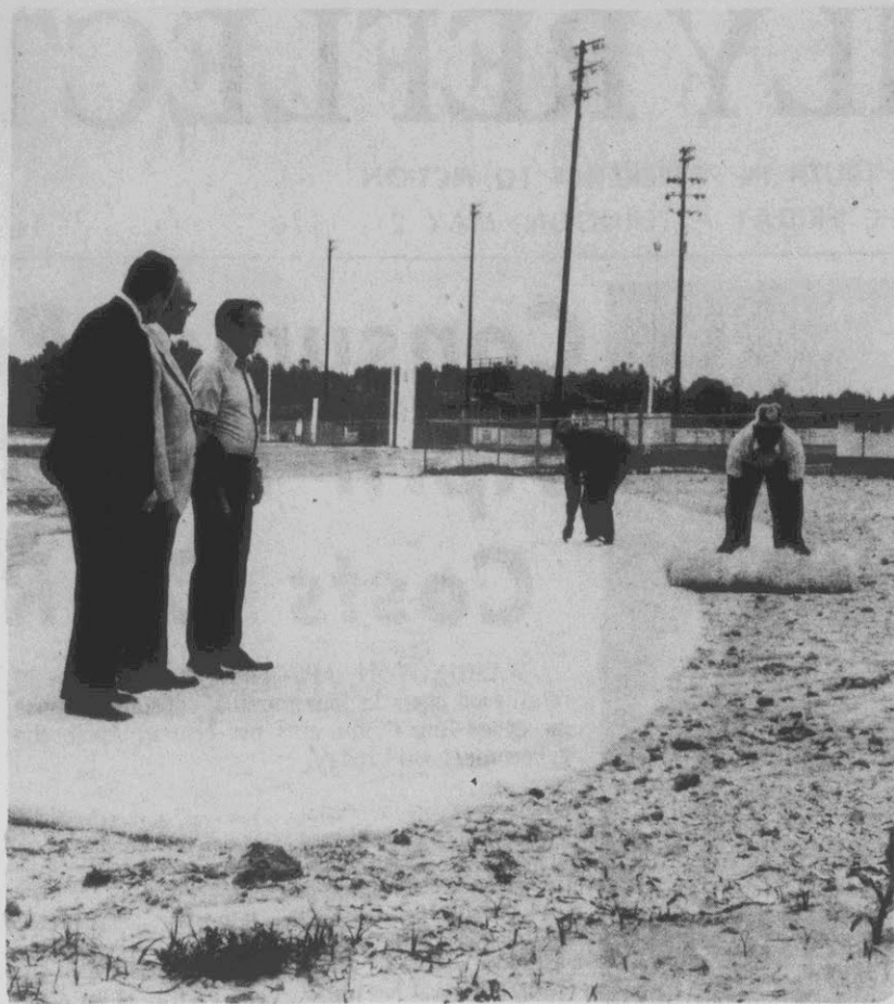
OBSERVE WORKMEN —Associate Superintendent of Pitt County Schools, Thomas Craft, left; Ralph Tucker of the Mid-East RC&D Council, middle; and Carl Heath, Maintenance
