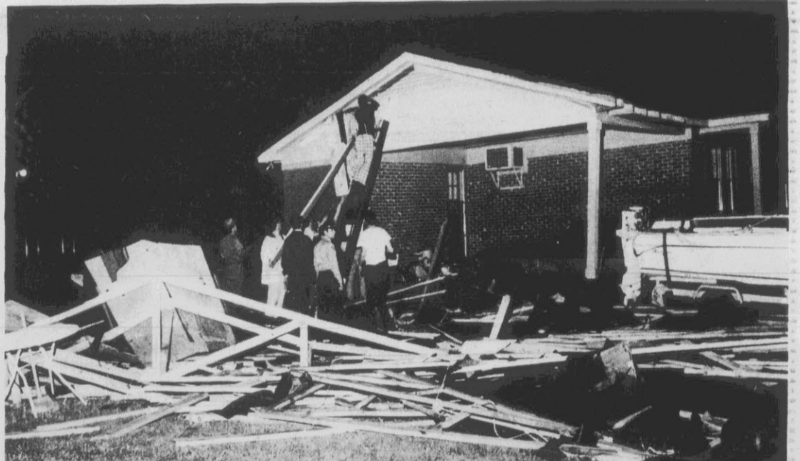
AFTERMATH OF HIGH WINDS . . . Neighbors and volunteers aid in the clean up after high winds damaged three homes near Winterville. (Reflector Photo by Tommy Forest)
