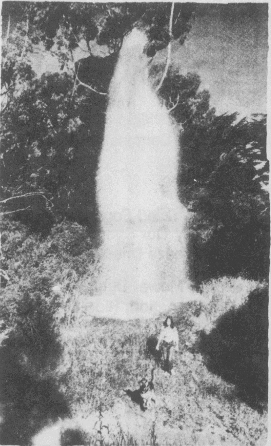
GOLDEN GATE GUSHER —Judy Handley walks her dog near a spouting water main in San Francisco's Golden Gate Park, which cut water pressure sharply in the city's Richmond District Tuesday. City officials said they suspected sabotage in the break of the 30-inch main which sent water 50 feet into the air, on the 28th day of a strike by city workers. (AP Wirephoto)
