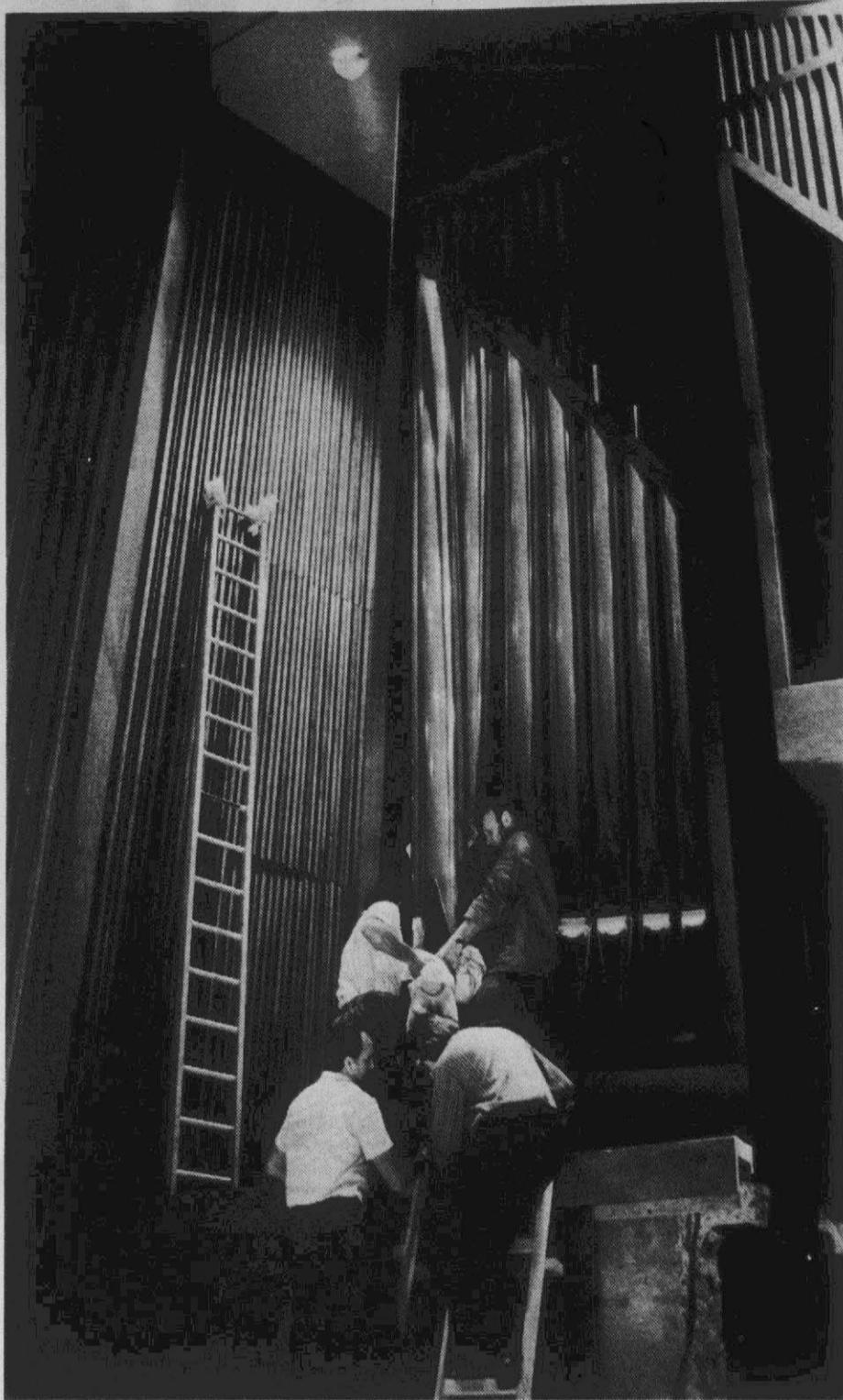
Sixteen-foot pipes are put in place in facade of organ.
