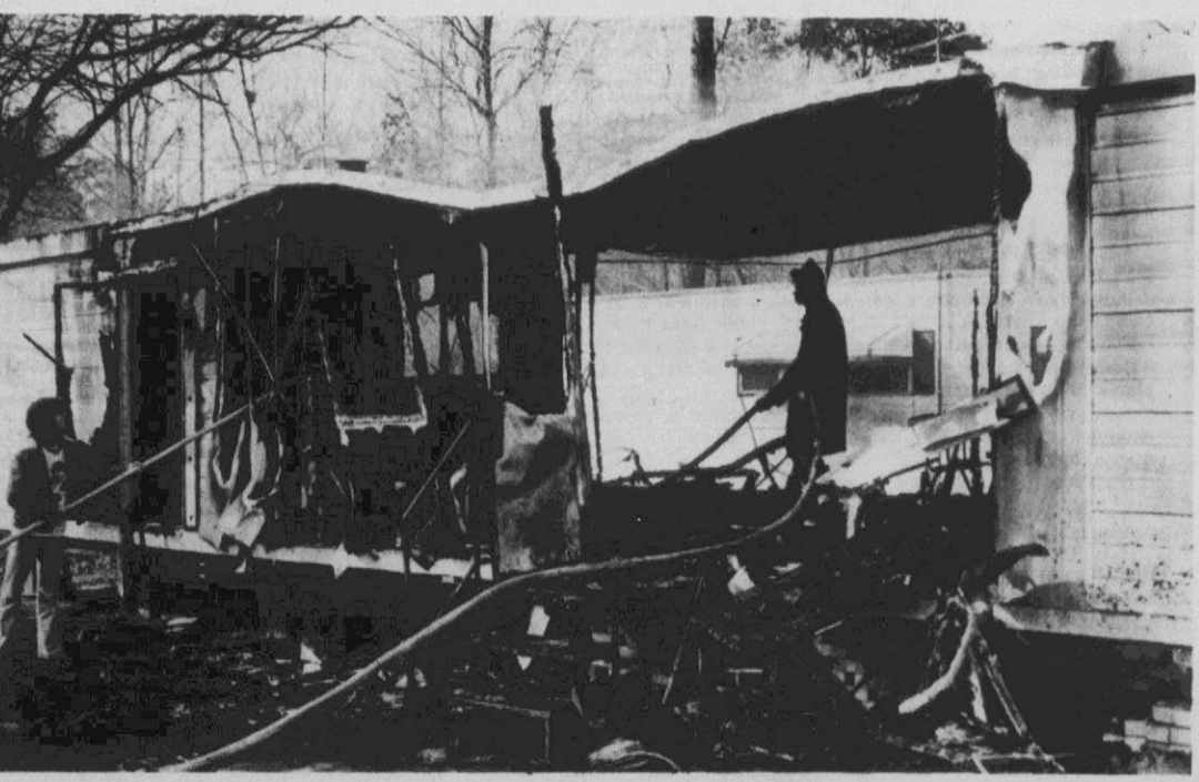
Flames Destroyed Mobile Home FIRE INJURES TWO — A mobile home fire at Azalea Gardens Trailer Park yesterday injured two workmen as they installed carpet. According to Pitt County Fire Marshal Bobby Joyner, the two injured were identified as Fountain Lewis McLawhorn, and John David McLawhorn employed by Whitehurst Floor & Carpet Center of Greenville. Joyner said a gallon of contact cement was dropped when there was a flash fire causing both men to be burned. The mobile home was completely destroyed in the 1:45 p.m. alarm. Members of the Eastern Pines Fire department responded to the call. (Reflector Photo by Tommy Forrest)
