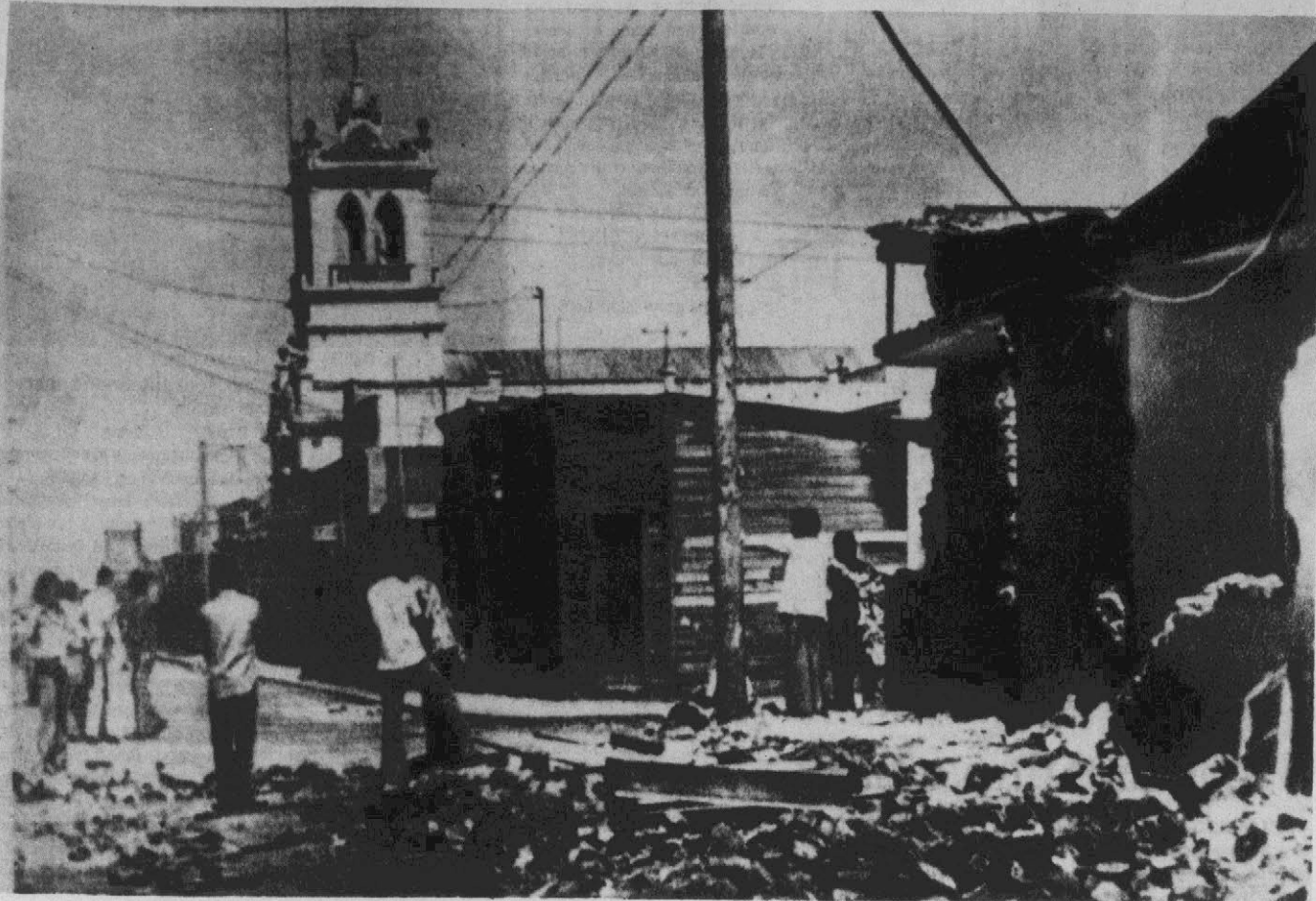
STILL STANDS—This church in the center of Guatemala City withstood Wednesday morning's powerful earthquake, which killed perhaps as many as 2,000 persons. Local residents stand amidst the rubble of smaller buildings in the foreground. (AP Wirephoto)
