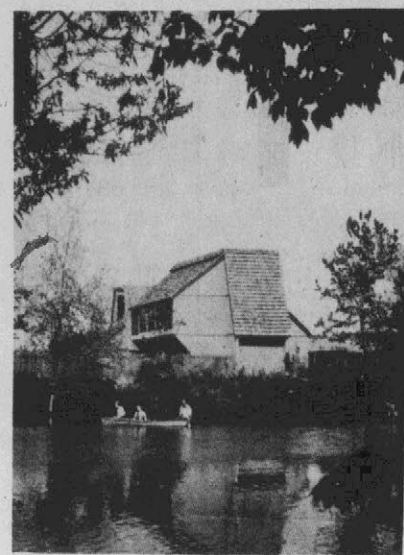
View of the Recreation Complex from across the lake.
