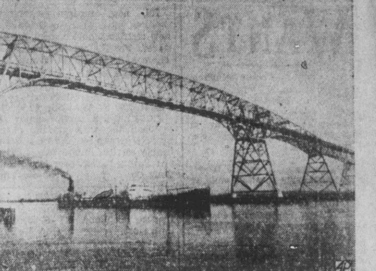
TALL TALES IN TEXAS concern above $2,750,000 span—one of the south's tallest highway bridges, to be opened to traffic in September. The toll-free bridge, crossing the Neches river at Orange and Port Arthur, towers 230 feet above the water, at its highest point. The main span provides a clearance of 176 feet above water. Structure is 1 1/2 miles long.
