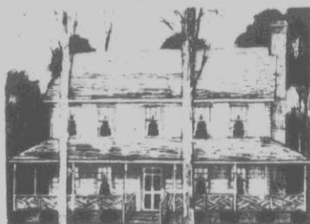
Category 4 CARTRETTE CONSTRUCTION CO. Cherry Oaks
