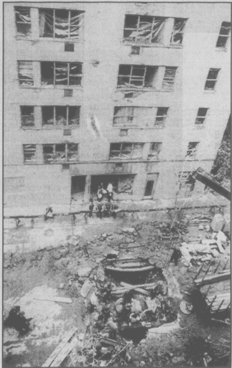
A crew works Sunday to repair steam pipe in Manhattan
