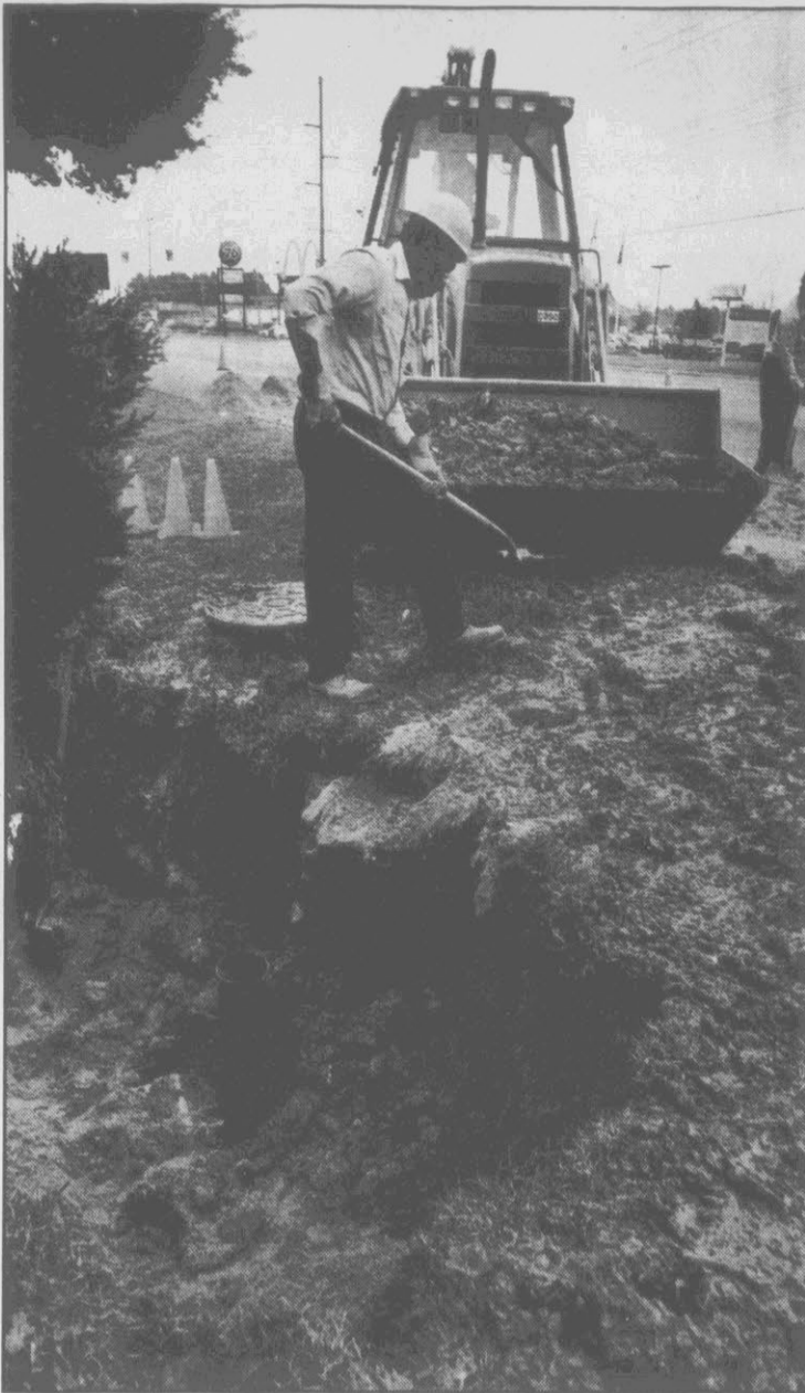
Joseph Shelley works in area where gas leak developed
