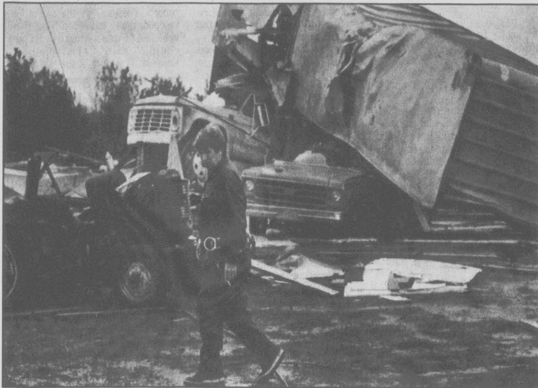
Fletcher Lee of Morven looks over damage caused by tornadic winds to his cable TV plant
