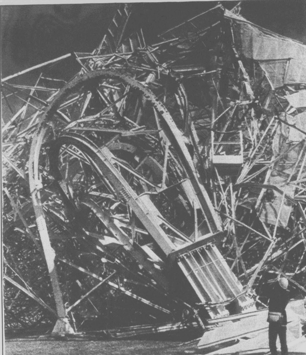
Debris from a 300-foot diameter telescope lies crumpled at Green Bank, W.Va., observatory
