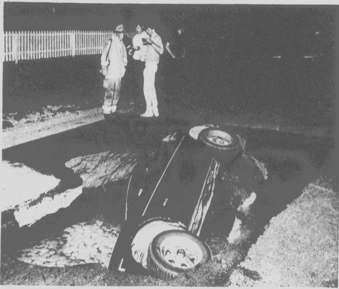
BIG POTHOLE — Erosion following a sewer project caused a street in Salisbury to cave in Thursday when motorist Michael Kendrick drove his car into what appeared to be a small pothole. When the car struck the little hole, the pavement collapsed, plunging the vehicle into the opening. (AP Laserphoto)
