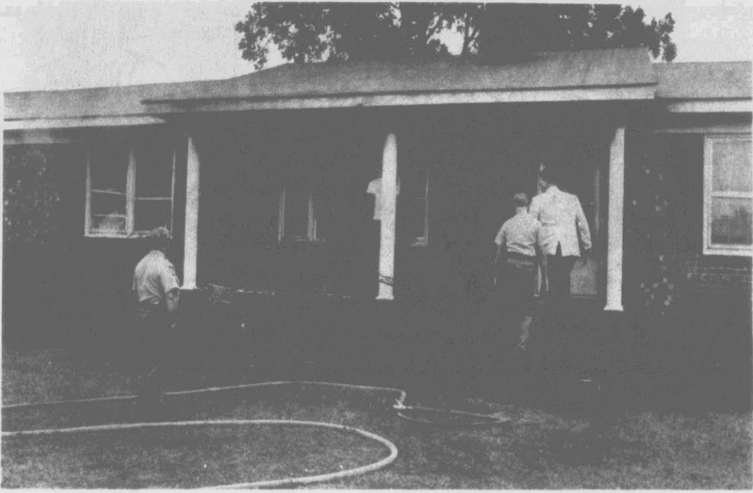
FIRE FACILITY — Fire investigators look over a home on secondary road 1772 near Hudson's Crossroads early this morning after fire claimed the life of Robert Lee Edwards Jr. According to Pitt County Fire Marshal Bobby Joyner, the fire was discovered about 6:40 a.m. by Edwards' wife. Edwards was in the den of the home and
