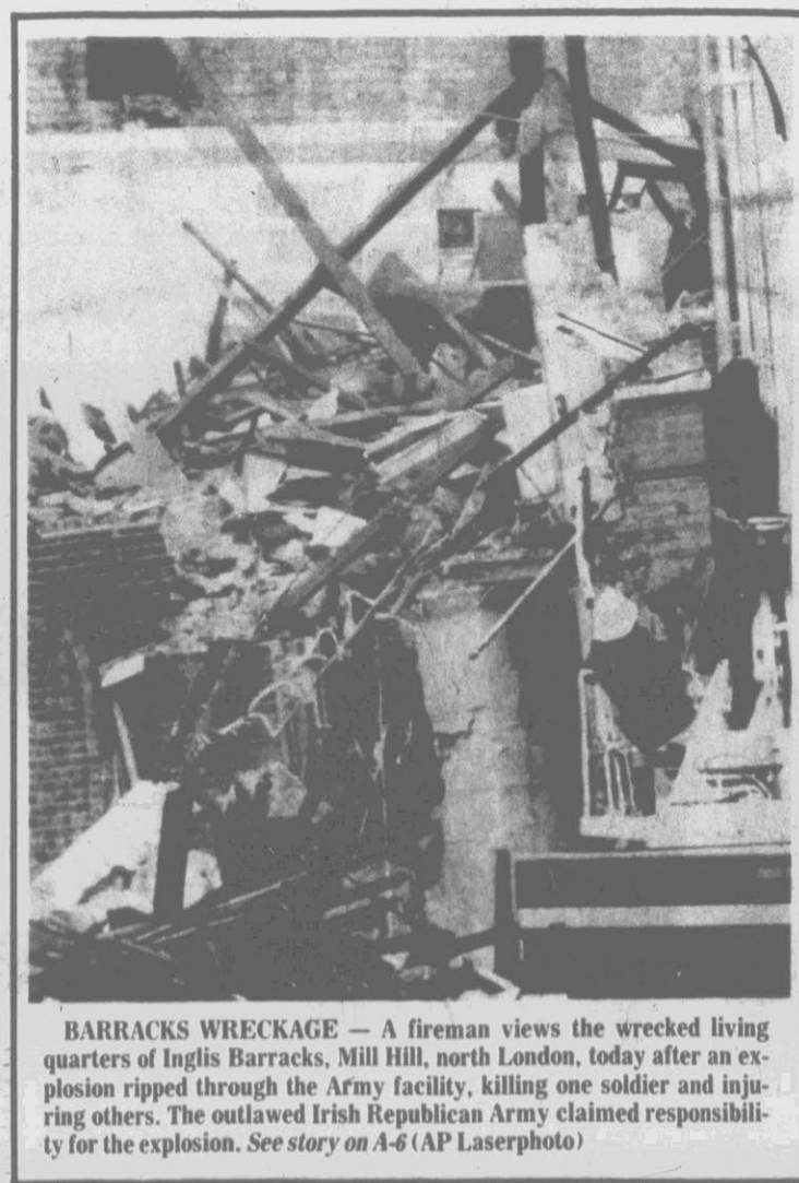
BARRACKS WRECKAGE — A fireman views the wrecked living quarters of Inglis Barracks, Mill Hill, north London, today after an explosion ripped through the Army facility, killing one soldier and injuring others. The outlawed Irish Republican Army claimed responsibility for the explosion. See story on A-6 (AP Laserphoto)
