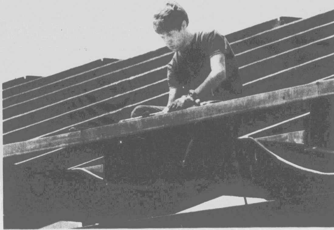
WORK IN THE RAFTERS —Louis Wallace does some welding Tuesday afternoon on the roof at Greenville Middle School. Scorching summer temperatures make outdoor jobs, especially roof work, kind of tough. (Reflector Photo by Cliff Hollis)
