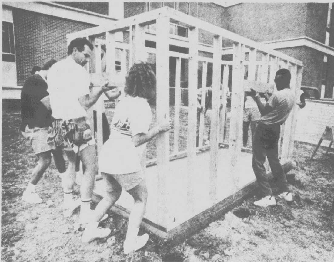
STORAGE FOR TRICYCLES — Putting an assembled framework on a concrete foundation are construction management students at East Carolina University who completed the new playground facilities project for
