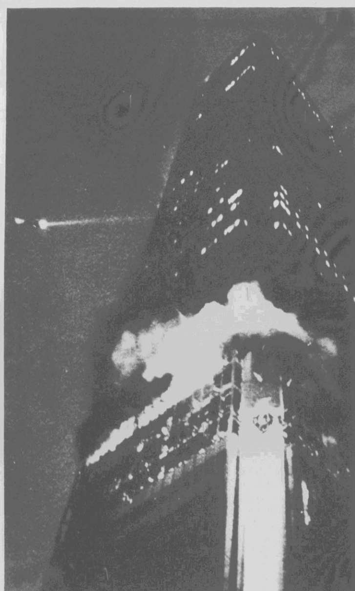
TOWERING FIRE — A fire department helicopter at left flies around the First Interstate Bank Building in Los Angeles early today as fire shot from the windows of the 62-story building. One man trapped in an elevator was killed and more than 30 others were injured before the fire was put out. See story on A-12. (AP Laserphoto)
