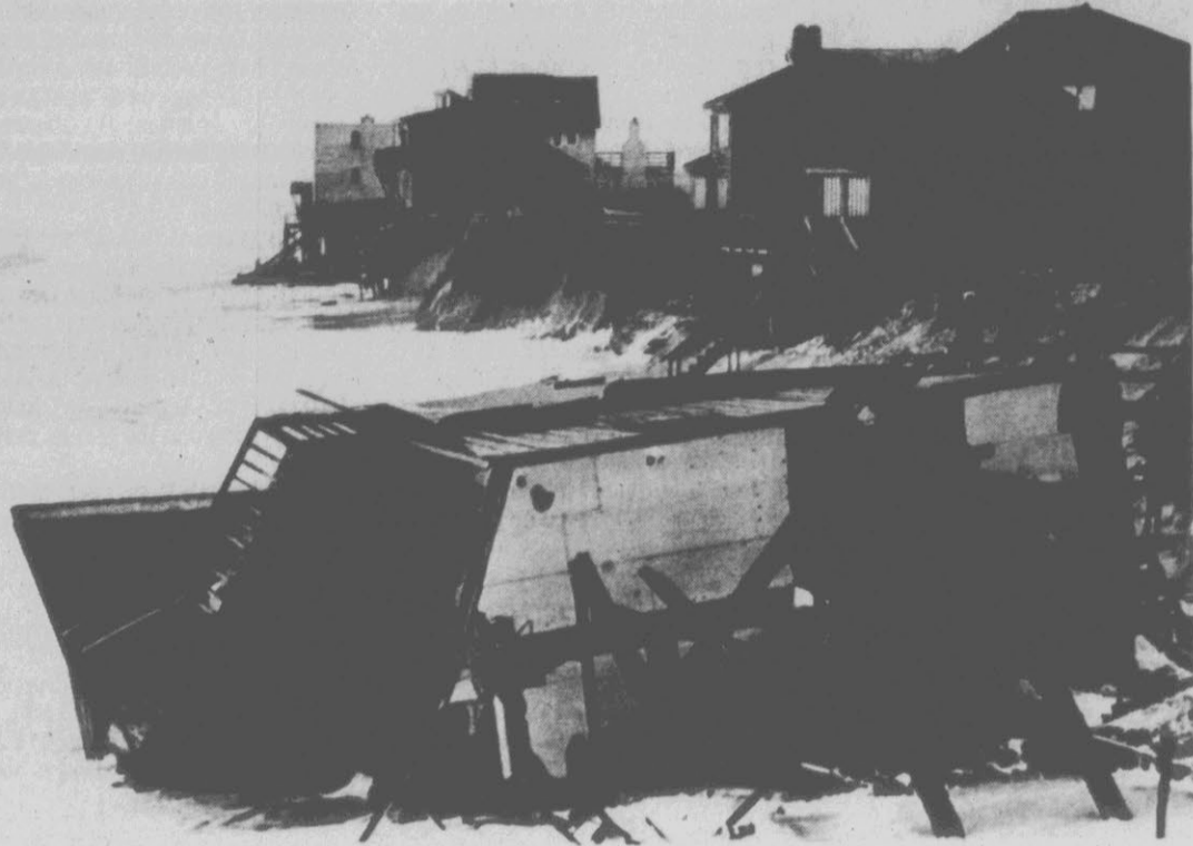
COASTAL DAMAGE — An oceanfront cottage, condemned earlier because of erosion, rests in a crumpled heap after it collapsed at Nags Head Wednesday evening as a northeaster pounded the coast with hurricane-force winds. Wind-swept tides caused heavy erosion at Oregon Inlet, threatening the Herbert C. Bonner Bridge. (AP Laserphoto)
