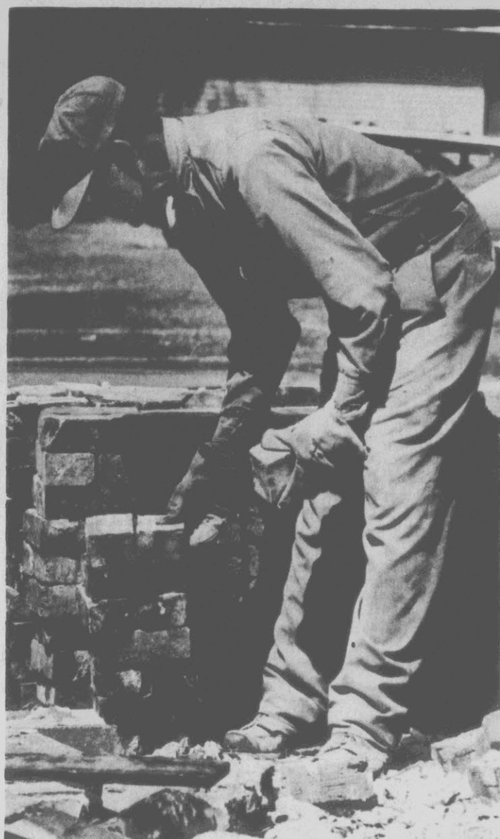
RECOVERING BRICKS — Pete Valentine stacks bricks at the corner of Evans and 13th streets Wednesday. He was recovering old bricks from a house that had been torn down. He said the bricks would be used in other chimneys and fireplaces. (Reflector Photo by Cliff Hollis)
