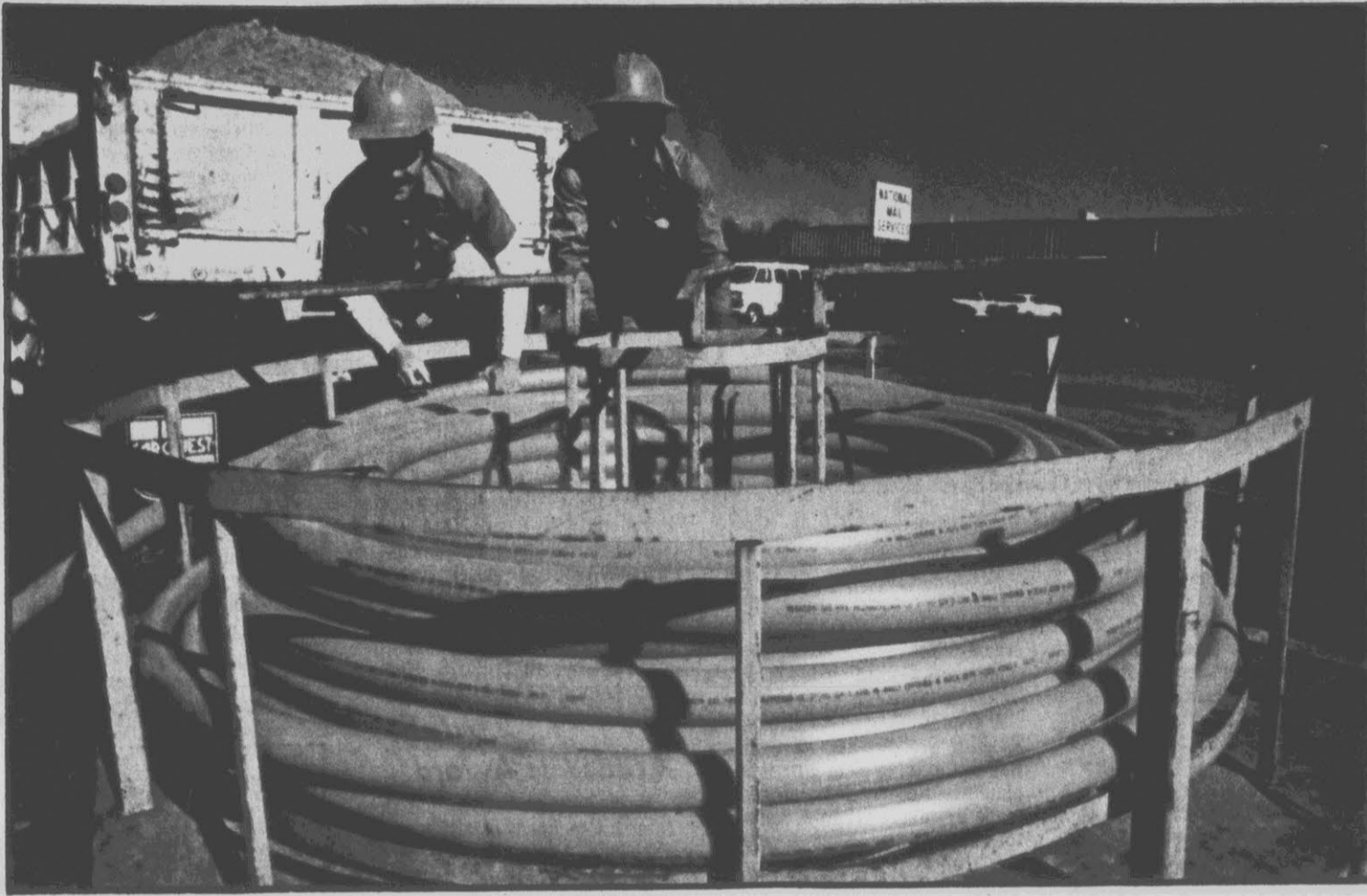
COLORFUL PIPE — Greenville Utilities gas department workers Allen Nethercutt, left, and Robert Cox work with large two-inch orange gas pipe to be placed under Evans Street Tuesday. The gas line is an extension of the main feeder line serving a nearby shopping center. (Reflector Photo by Thomas Forrest)
