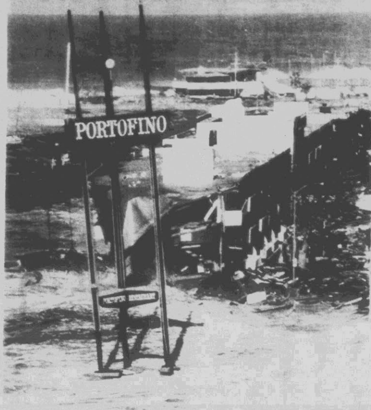
DAMAGED COAST — Waves smash into the Portofino Inn at Redondo Beach, Calif., Monday after a winter storm pushed through the area. Several buildings were damaged and a state of emergency was called by city officials. (AP Laserphoto)
