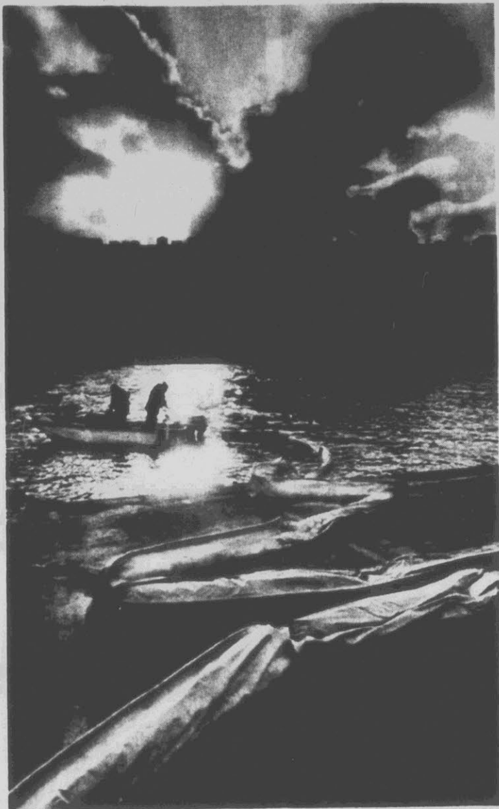
RIVER CLEANUP — Workmen drag a boom late Monday into the Monongahela River as part of the cleanup of a million gallons of diesel fuel that spilled when a storage tank collapsed. Thousands of people in the Pittsburgh area have been forced to ration water during the cleanup. See story on A-3. (AP Laserphoto)
