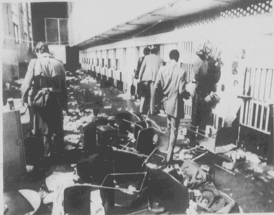
DAMAGED CELLBLOCK — Members of a press pool step over debris as they tour cellblock C at the U.S. Penitentiary in Atlanta Wednesday. Cuban inmates took over the prison for 11 days in protest of U.S. plans to send some refugees back to their homeland. (AP Laserphoto)
