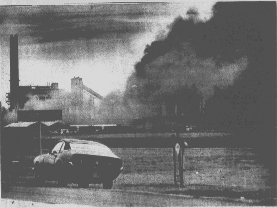
PLANT EXPLOSION — Smoke pours from a Celanese chemical plant in Pampa, Texas, Sunday after two explosions heavily damaged the facility. Three workers were killed. (AP Laserphoto)
