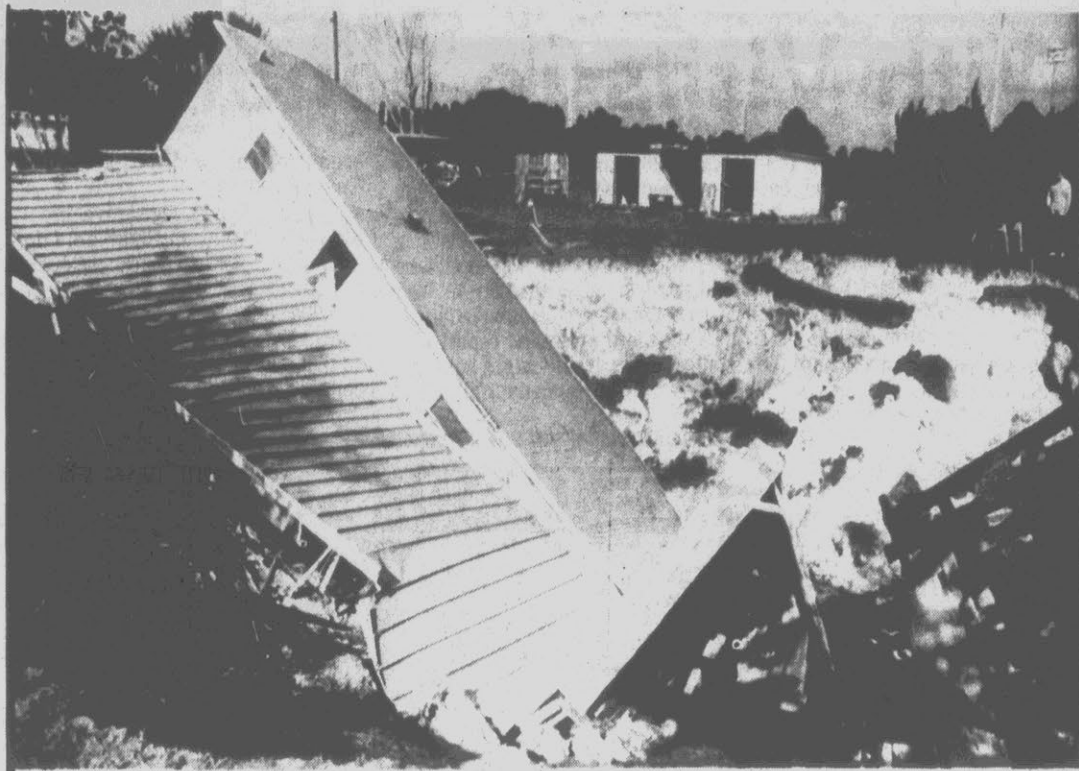
SINKHOLE — A sinkhole gobbles up a 60-foot mobile home Wednesday in Odessa, Fla. Six persons in the home escaped without injury when the hole began opening
