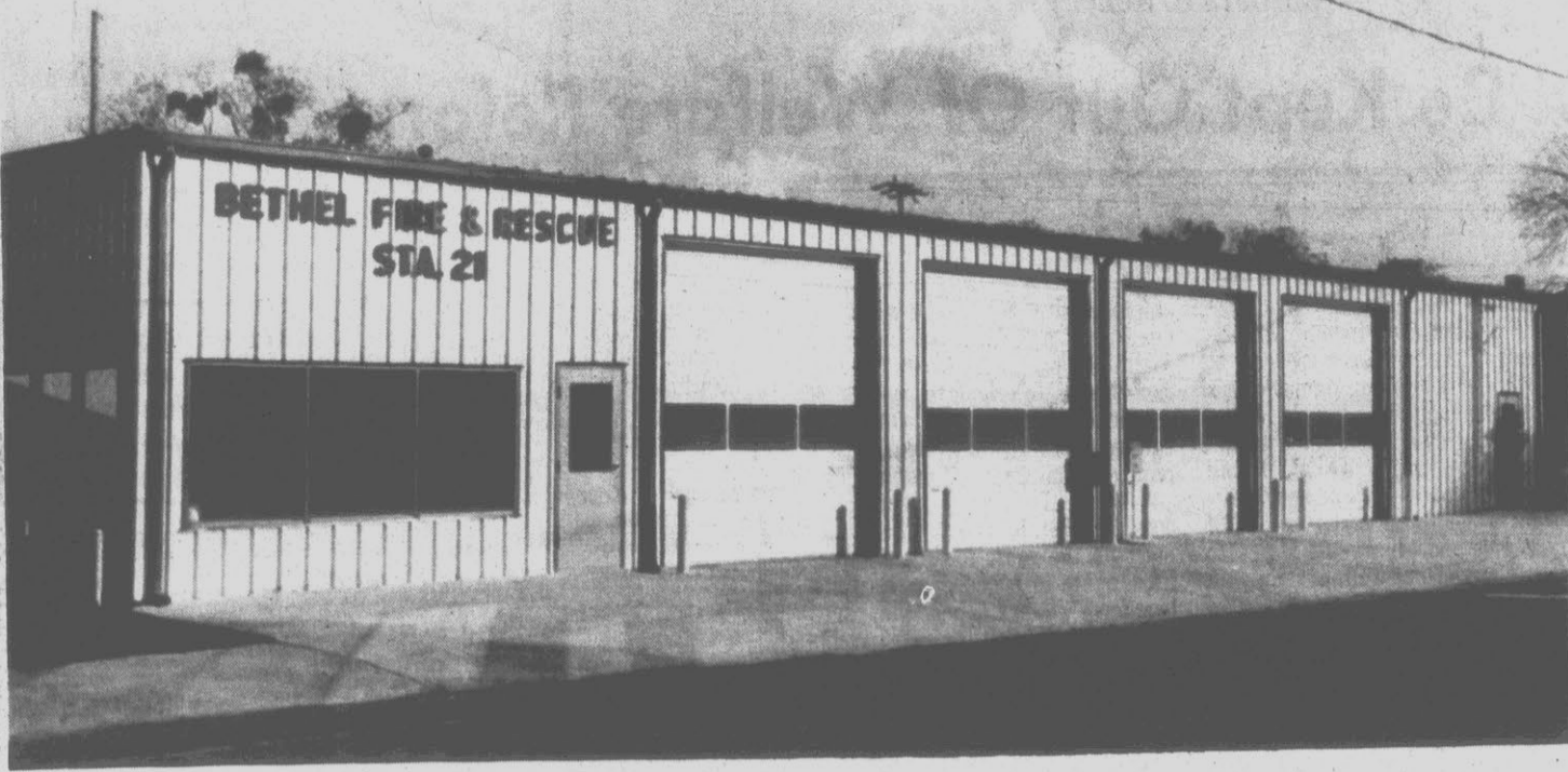
NEW FACILITY — A new fire and rescue building has been constructed in Bethel. The 6,000 square-foot facility has eight bays and can house 11 fire and rescue trucks. The building project was begun in November 1986 and was completed last month. An open house will be held Sunday from 2-5 p.m. The
