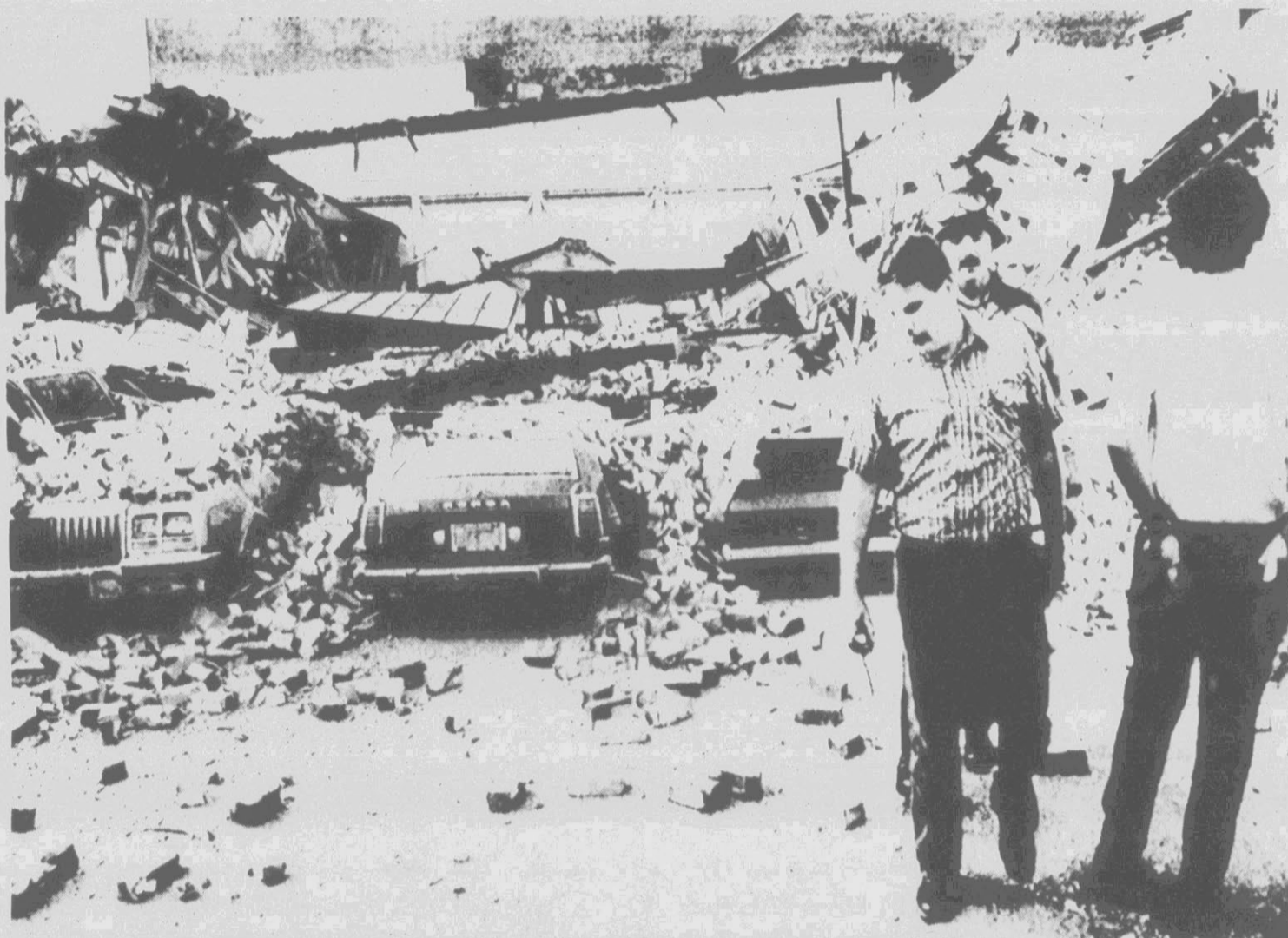
QUAKE DAMAGE — Pasadena, Calif., officials look at some of the wreckage left by Thursday's major earthquake. The quake, which registered 6.1 on the Richter scale, caused the building shown here to collapse, crushing
